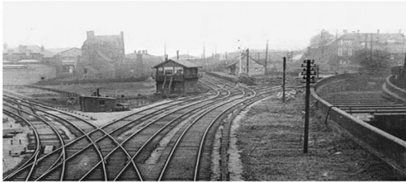
Looking east toward Connaught Road Station. Beckton branch diverges left & North Woolwich diverges right. The later deviation leading to Connaught Tunnel is shown on the extreme right.
